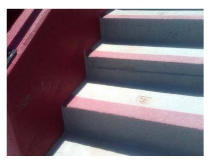
f. Joint System Schedule; EJ Type "F" – Add the following to the joint description: "Contractor is to mask both sides of the joint when applying the 3/8"urethane sealant topping in order to ensure a clean and consistent joint condition".
